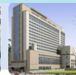
Kokilaben Dhirubhai Ambani Hospital and Medical Research Center
